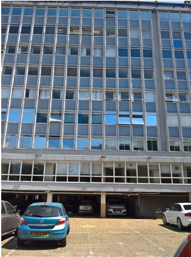
Rear elevation, rear tower building
