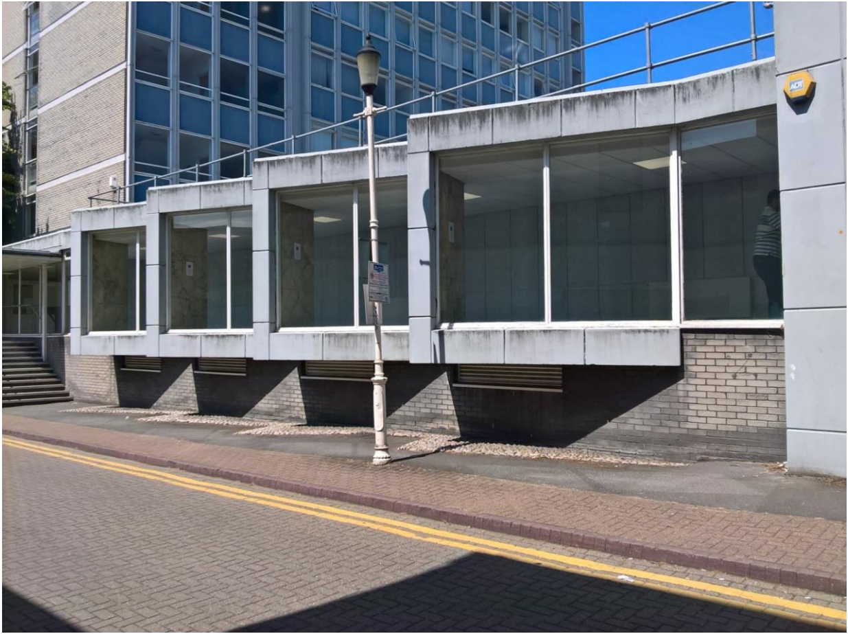
Raised ground floor and front elevation of the rear tower, viewed from south on Spring Villa Road
