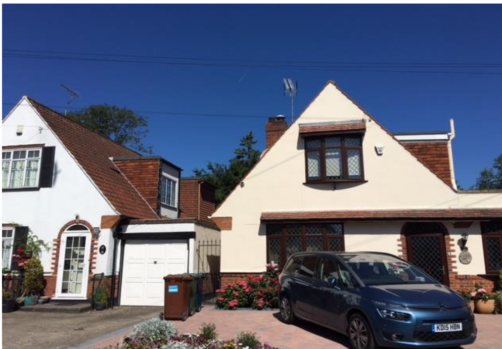
Photo showing front elevation of No.5 Wynlie Gardens (Left) and No.3 Wynlie Gardens (Right)
